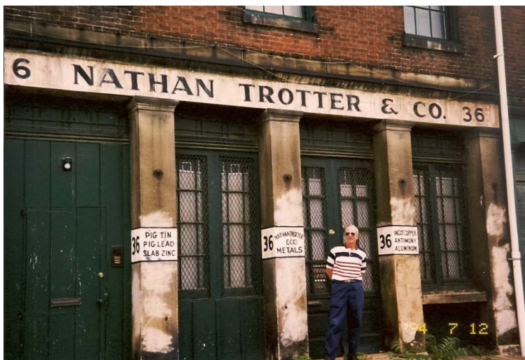
Fig. 1: Nathan Trotter & Company historic façade.
